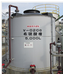
As the picture shows, our displays allow workers to recognize the hazardous nature of chemicals that give rise to exposure concerns.
