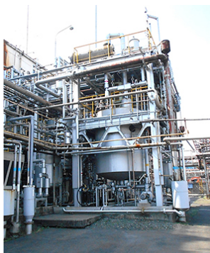
Distillation Recovery Facility
