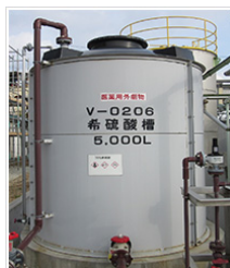
Workers are made aware of the hazards and toxicity of the chemical substances that they could be exposed to.
