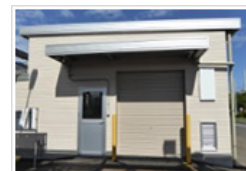
Pilot test facilities
