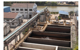
Wuxi Advanced Kayaku Chemical's wastewater treatment facility
