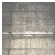
After construction with FLOWSEALER
