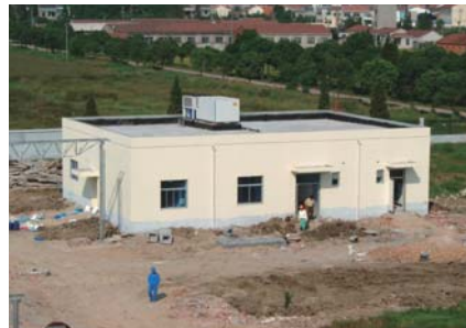
Plant of WPLC (China), a subsidiary of Polatechno, under construction
