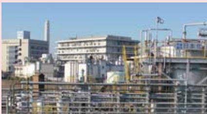
●Tokyo Plant ▶P41
