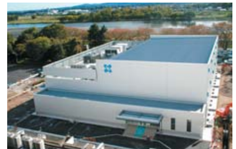
The 2nd formulating factory near completion
