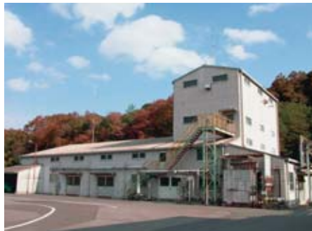
Slurried explosives factory
